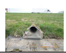
18 RCP from Northland Av curb inlets discharges to concrete channel from north. (Formerly SS-0-X4)
