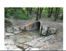
54 RCP discharges to riprap channel. Ultimately discharges through NN-1-X. (Formerly Y-266-X)
